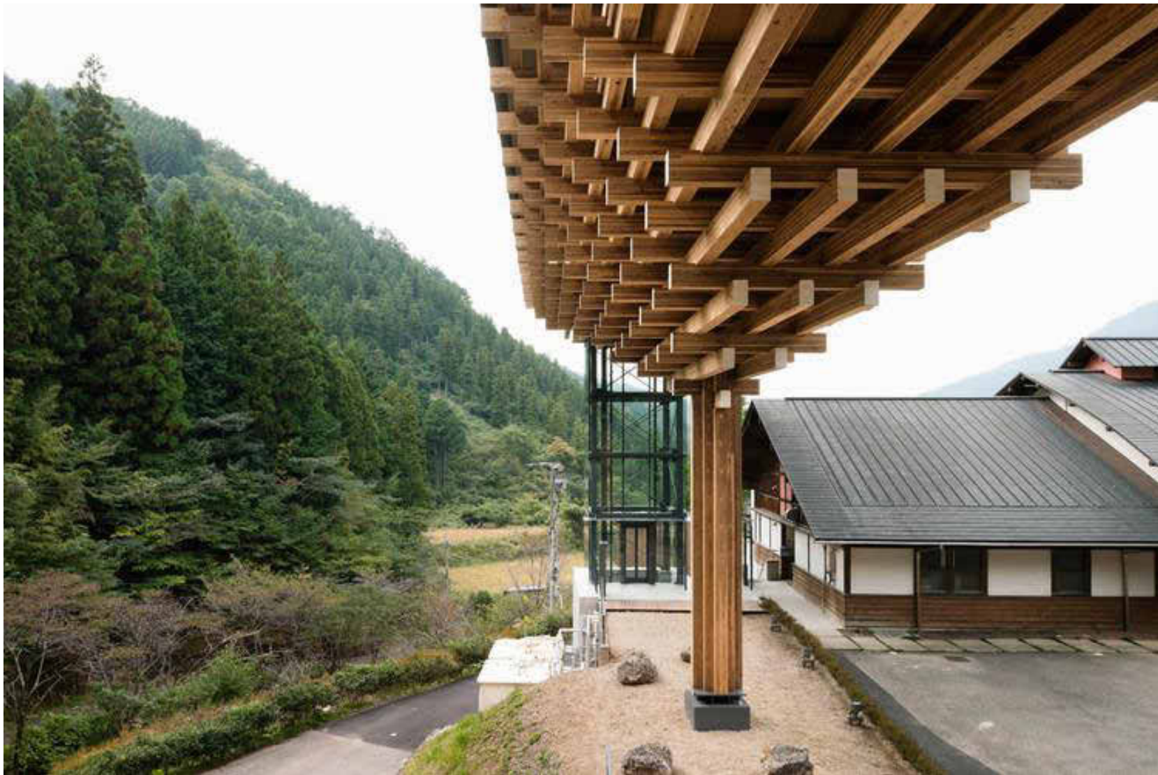
Yusuhara Wooden Bridge Museum — Kengo Kuma (2010), Japan. Cantilevered cedar bracket system (tokyō), timber cruciform structure.
