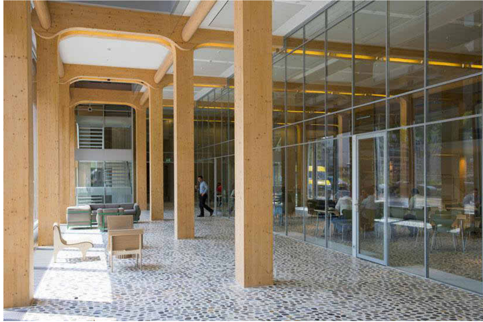
Tamedia Office Building — Shigeru Ban (2013), Zurich. All-timber moment frame, no metal fasteners, interlocking spruce joinery.
